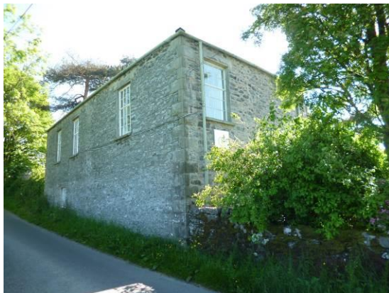
Fig.2: school room, now office, from the lane
